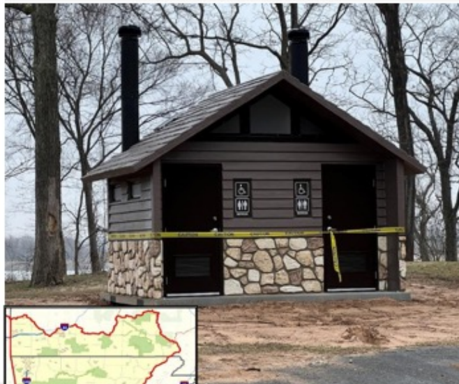
NEW RESTROOM AT DAMSITE 6 PARK
